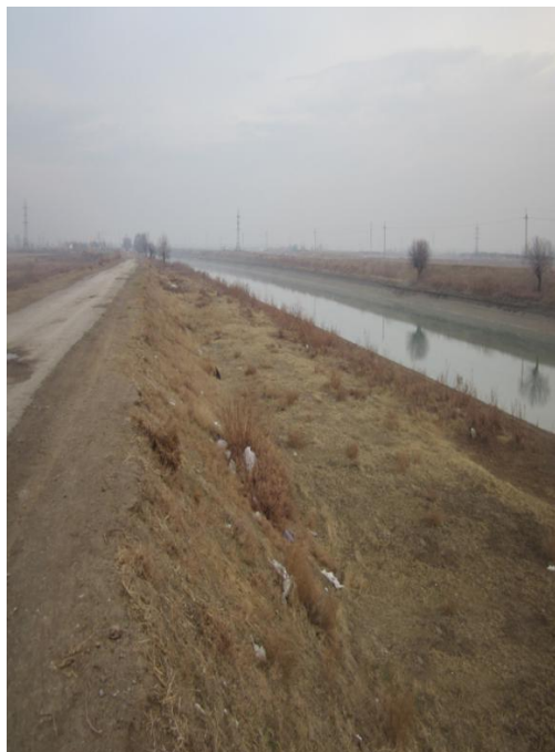
2-rasm. Qarshi magistral kanali PK700 dagi holat.
